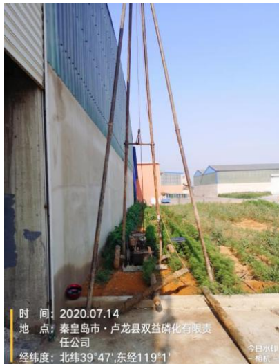
1I01/2I01 实际钻孔位置
